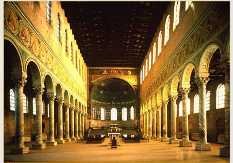
Nave looking towards the apse
